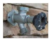
Here is a picture of an atmospheric vacuum breaker (AVB) installed on the bib.
